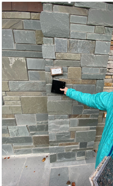
Pennsylvania Blue stone will be used for the walls
